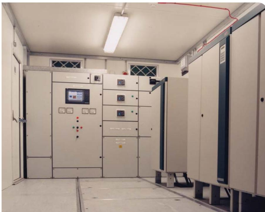
Category 'B' SPADs (Signals Passed At Danger) are the result of drivers passing signals when no aspect is showing. A national 650V UPS project was started to ensure that signal lamps and points remain operational should the power supply be interrupted.
